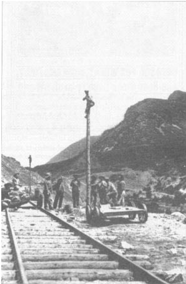
Fig. 3. Telegraph lines being erected on the Union Pacific near Ogden, Utah. ( Great American Railroad Stations , p. 9)
