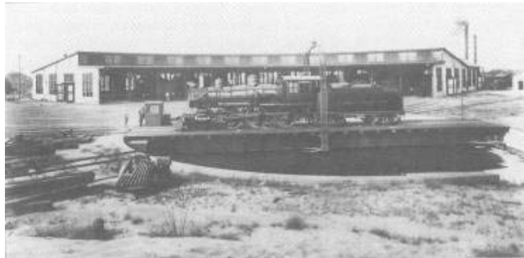
Fig. 1. Atlantic Coast Line roundhouse, Albany, Georgia, c. 1930. Note the monitor roof, which helped ventilate the building. (Great American Railroad Stations, p. 28)
